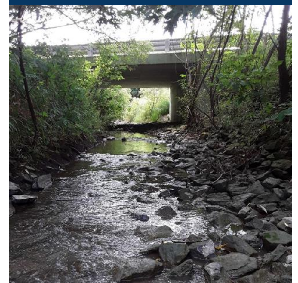
Lauzon Road Bridge over Little River Drain (Downstream)
