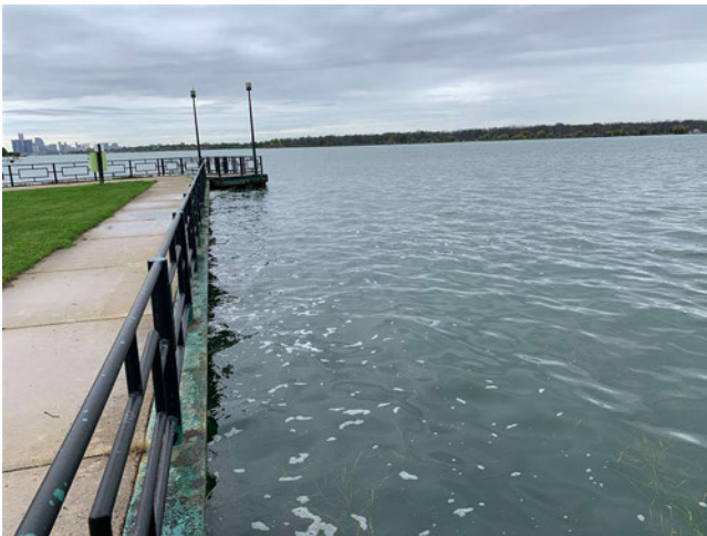
Photo 3: Conditions along the shoreline facing southwest. Date: October 18, 2021.
