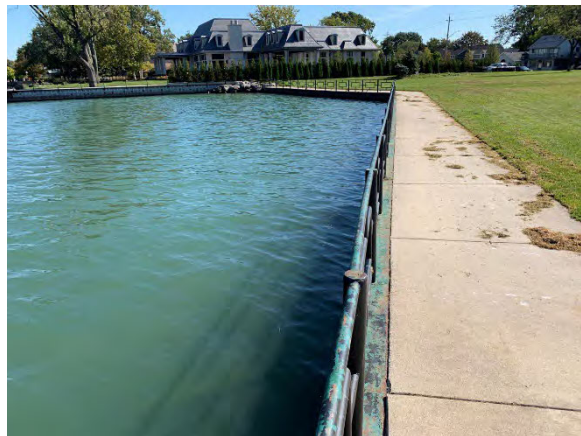
Photo 2: Showing retaining wall and portion of marine study area, facing southeast
