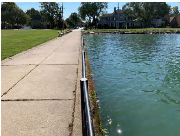
Photo 3: Showing retaining wall and portion of marine study area, facing south-southeast
