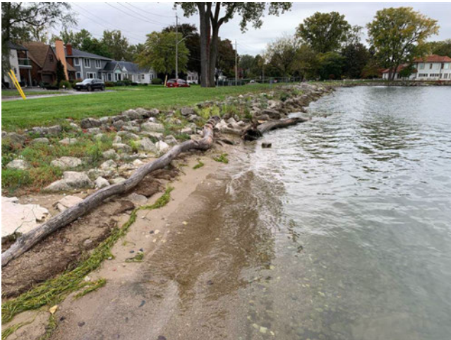
Photo 5: Conditions along the shoreline facing southwest. Date: October 18, 2021.
