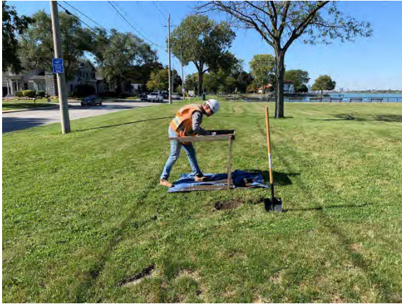
Photo 1: Test pit survey, facing southwest
