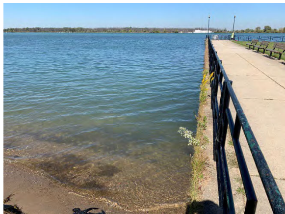
Photo 4: Showing retaining wall and portion of marine study area, facing north-northwest
