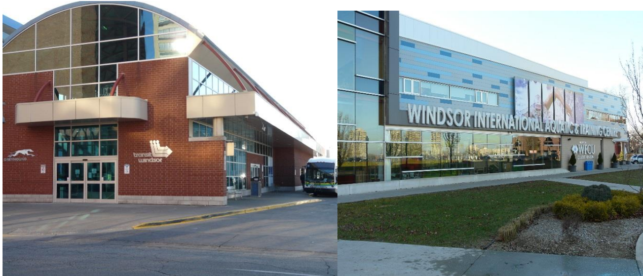
Overall Condition = Good
