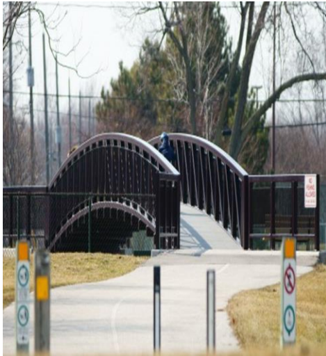
FIGURE 3-19—PREDESTRIAN BRIDGES CURRENT CONDITION LEVELS
