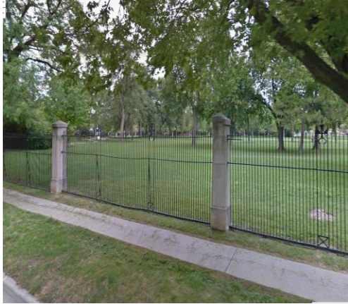
Overall Condition = Good
