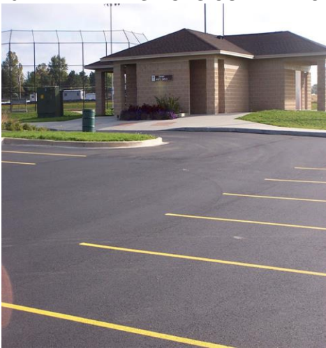
FIGURE 3-21—PARKING LOTS CURRENT CONDITION LEVELS
