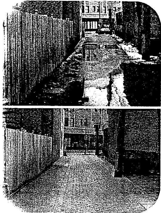
Figure 1: Stormwater runoff before (above) and after (below) porous pavement alley construction (Daley & Bryne, 2010)
