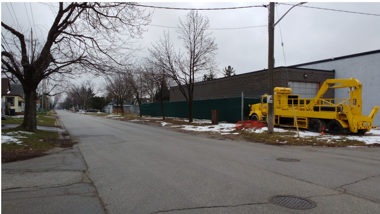
View of existing overhead door on applicant's property abutting south side of the area of closure
