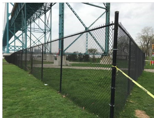
Coated chain link fence under Ambassador Bridge
