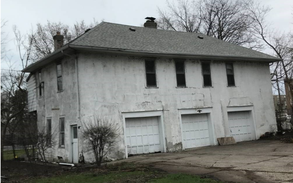
Garage, rear of 6425 Riverside Drive East, subject to request for demolition (2017)
