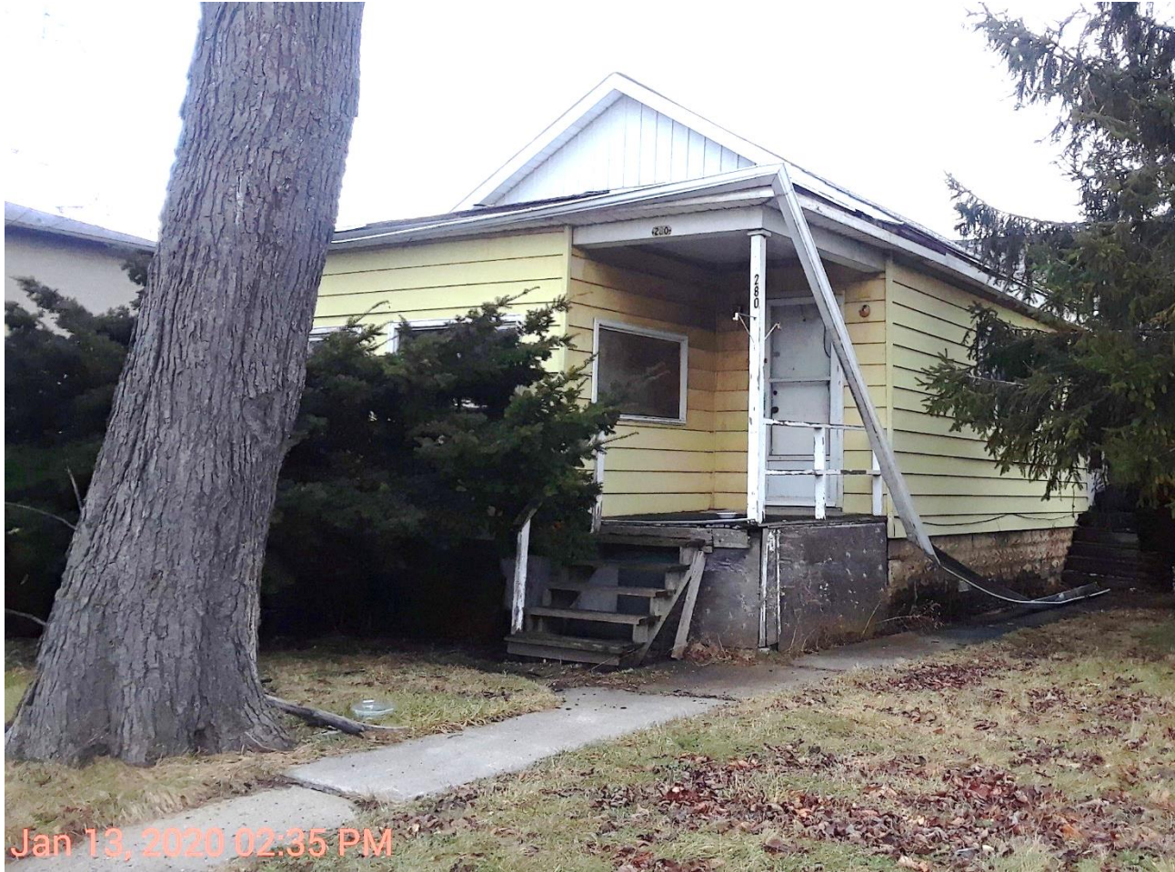
Front of building (West elevation)
