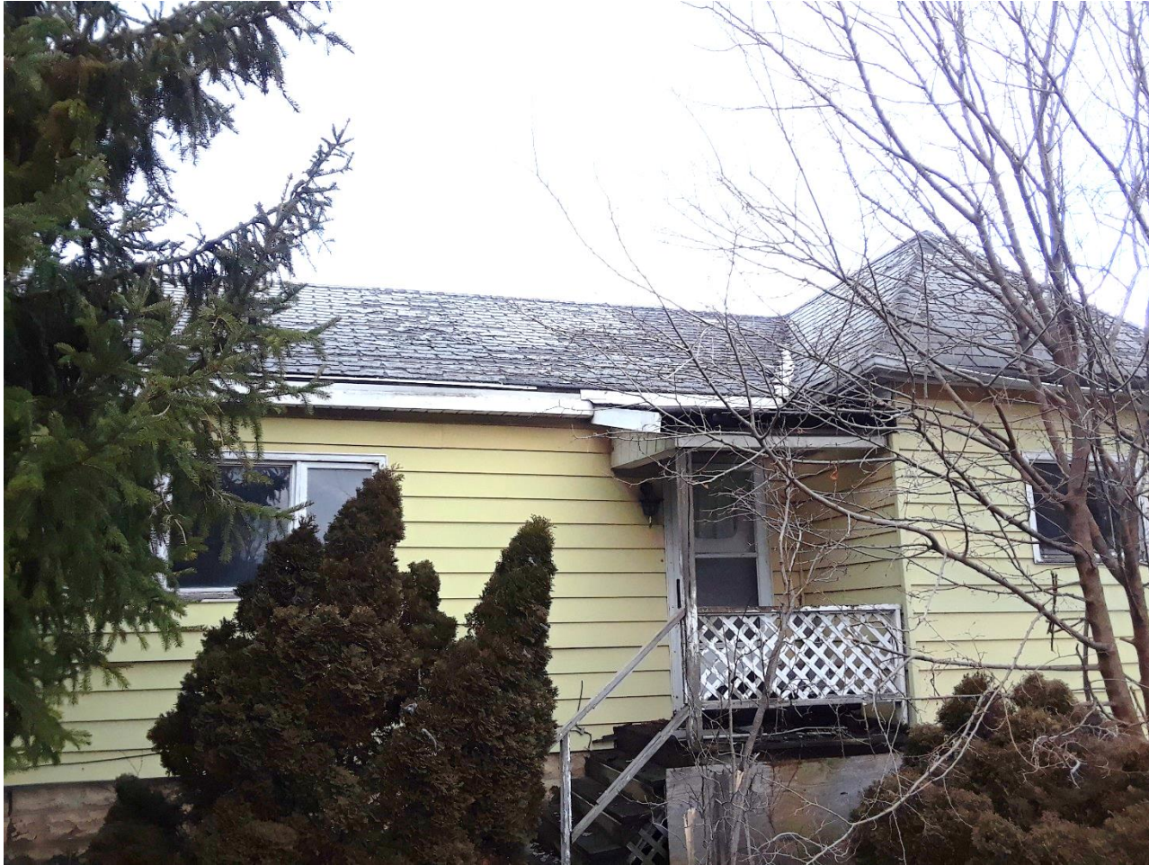
Side of building (South elevation)
