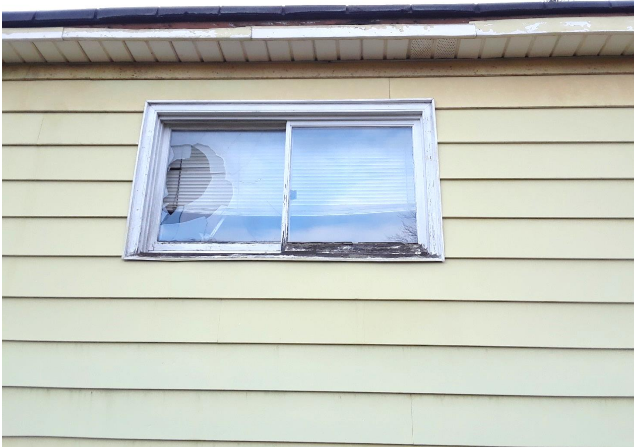
Side of building (North elevation)
