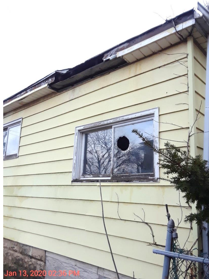
Side of building (North elevation)
