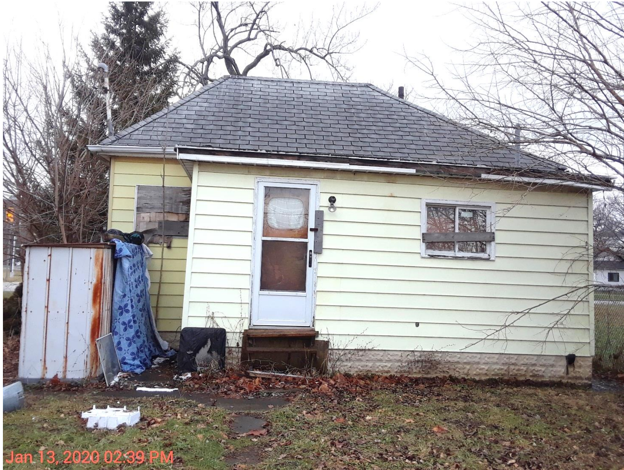
Rear of building (East elevation)
