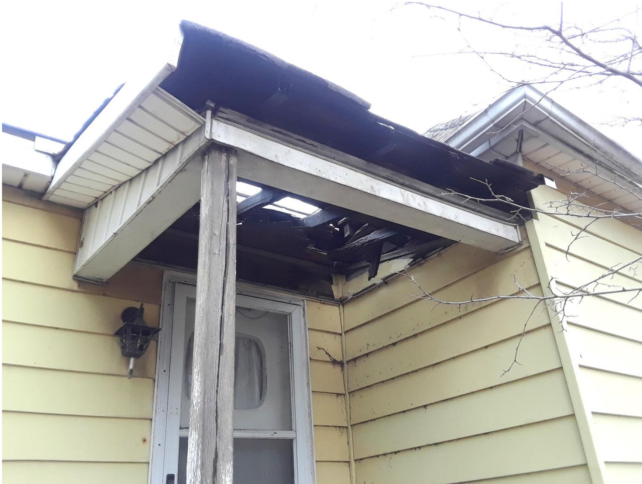
Side of building (South elevation)
