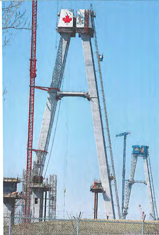
Work has begun on the support towers' final sections known as the pylonhead — the peak of the towers that will provide the support which feeds out the steel cables that will eventually hold up the bridge deck. DAN JARZBER
