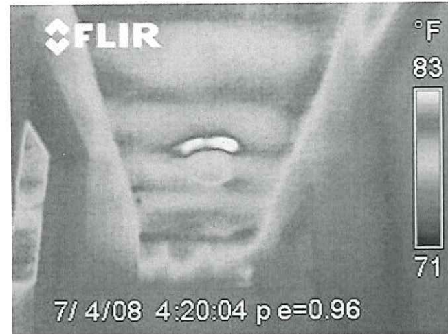
Here you can see the Infrared Image of the hallway. Because of poor insulation in the attic there is a lot of heat radiation to the inside of the house.
