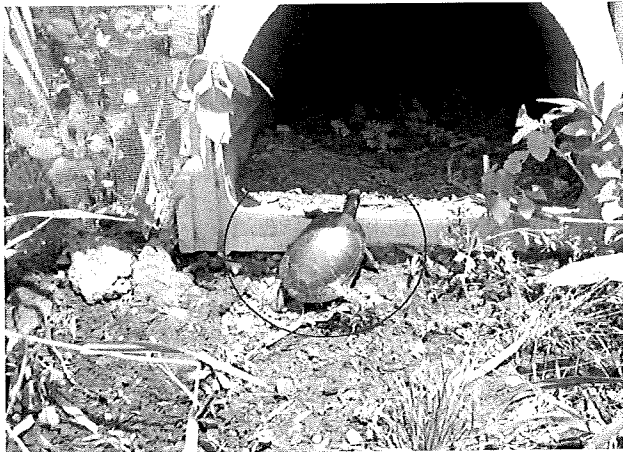
An eco passage seen in the Long Point Bay area (Photo courtesy of longpointcauseway.com)
