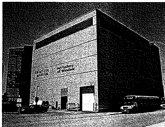
1F. South Side. Parking/ Street View. • LED Channel Lettered Sign. - New Hardware & Lighting.
