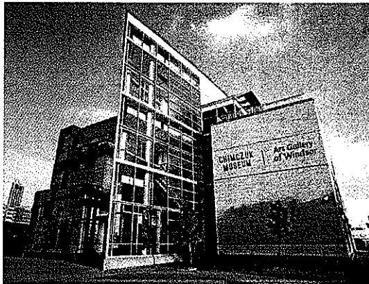
1E. North Side. Riverside View. • LED Channel Lettered Sign. - New Hardware & Lighting.
